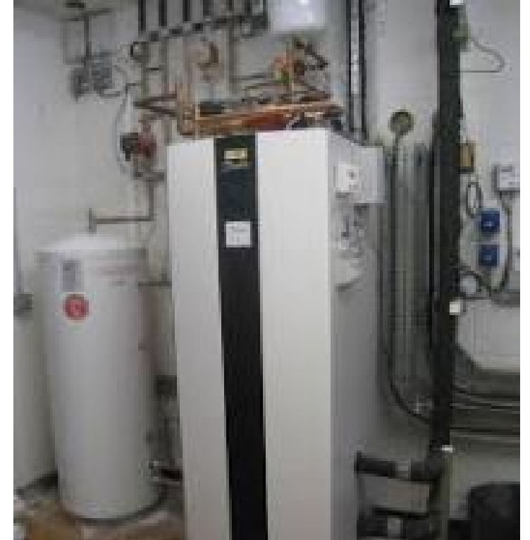
Heat pump at Dawdon Mine Water Treatments Scheme
