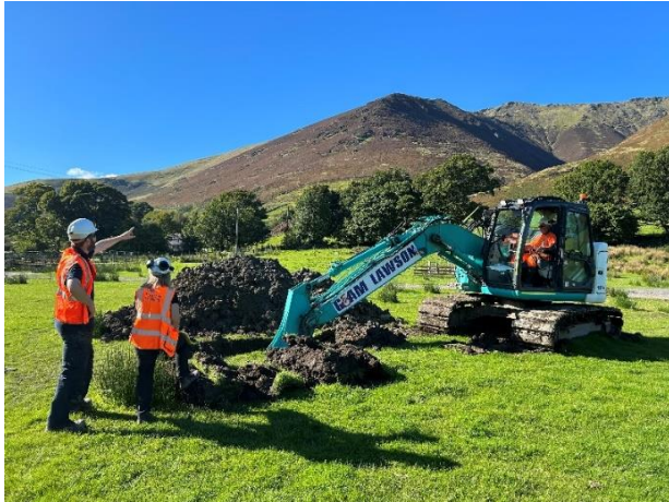
Photograph of a trial pit being dug.
