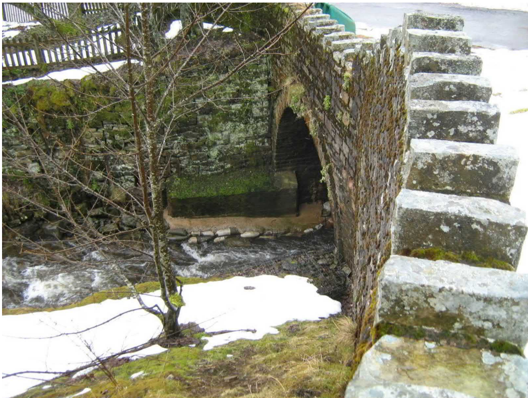
Plate 8. Culvert of the River Nent (TN1).
