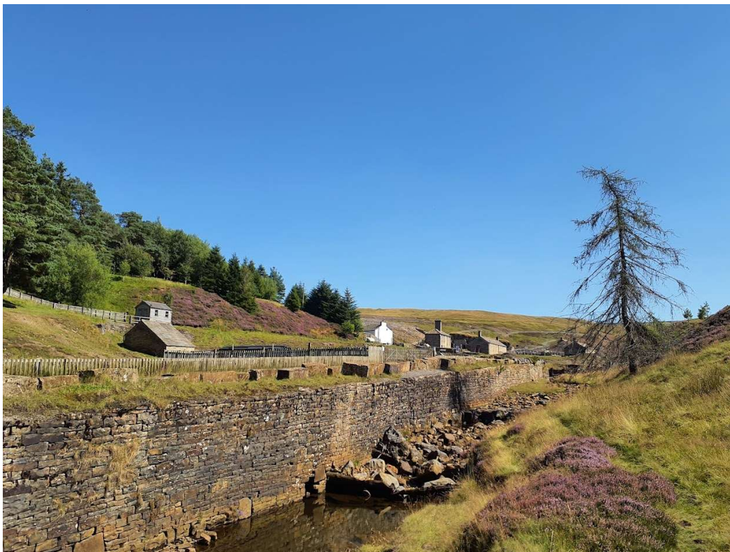
Photo 4 Looking southeast beyond T5
