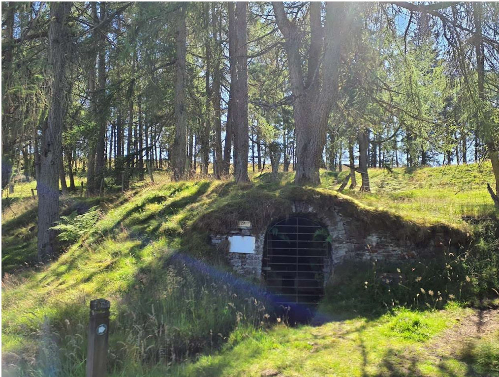
Photo 7 View of Caplecleugh adit with G14 behind
