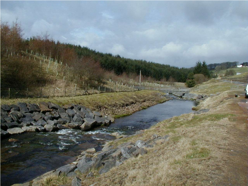
River Nent down stream of Nenthead Town (N4), weirs and gabions.
