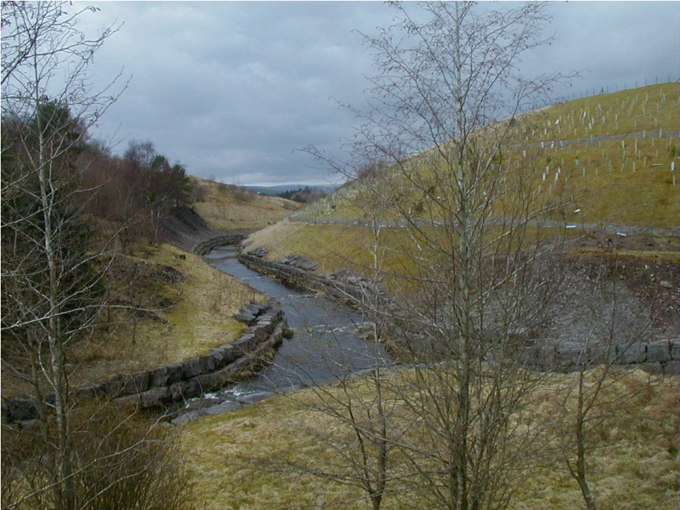
Brownley Hill tailings dam
