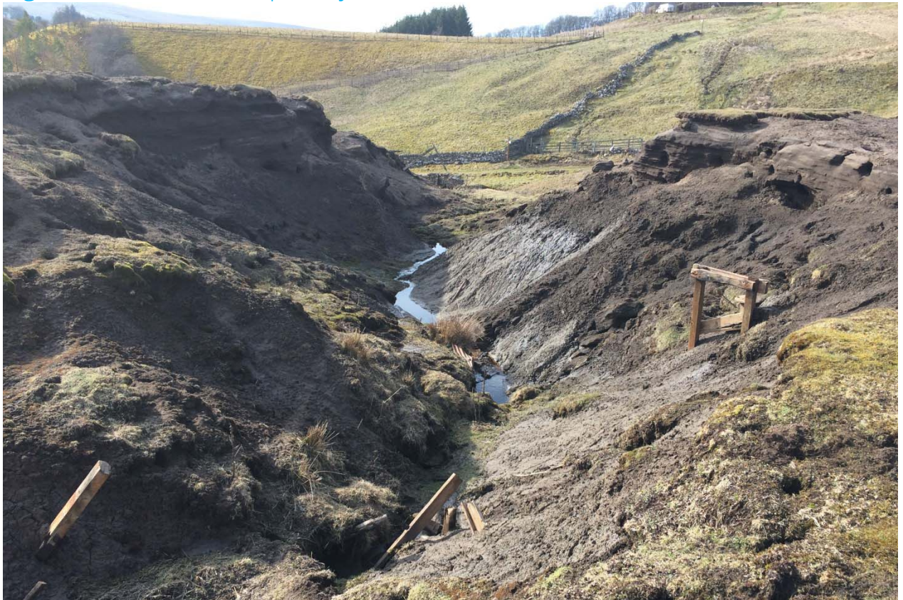
Figure 3.3 Eroded Deep Gully to Gudham Gill
